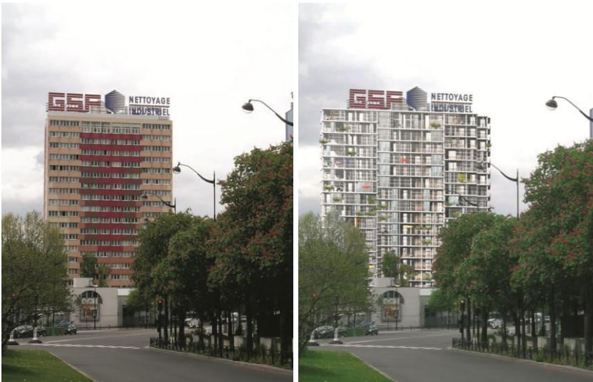
Bois-le-Prêtre Tower – BEFORE and AFTER. Rendering by Lacaton & Vassal Architectes.
