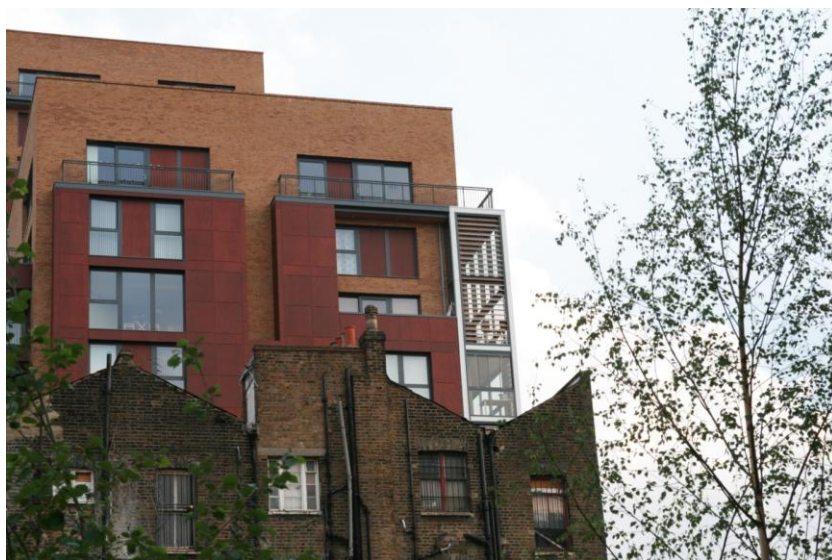
The Dalston Mill – View from the site to the new developments above the Dalston Junction Station. Ph: Author
