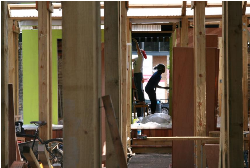
Dalston Barn – Apprentices and volunteers at work. Ph. below: Author
