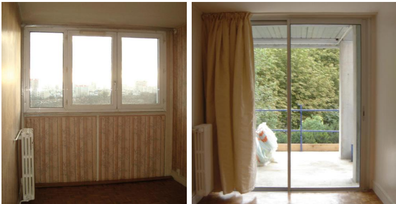
Bois-le-Prêtre Tower – Installing a prototype: BEFORE and AFTER
