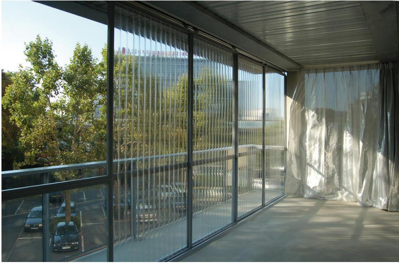
Bois-le-Prêtre Tower : Apartment interiors photographed and registered by Lacaton & Vassal Architectes. Interiors could be kept unchanged while winter gardens and terraces were added.
