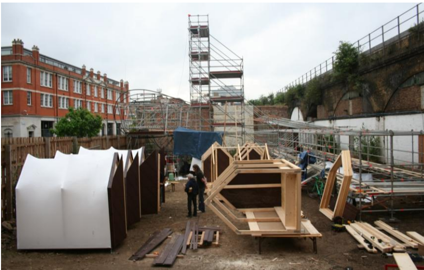
Southwark Lido – Constructing beach huts. Source: Exyzt
